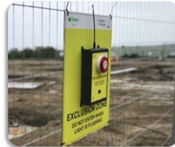
Full physical segregation
